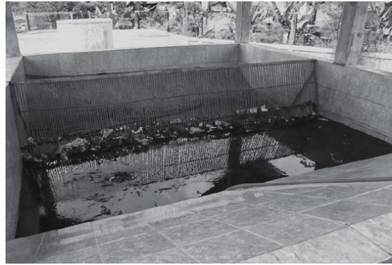
Figure 47: Enclosed Screen With Potential Hazard of Gases
