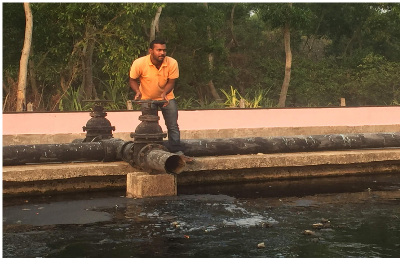
Figure 54: Poor Access to Tanks, Beds and Valves
