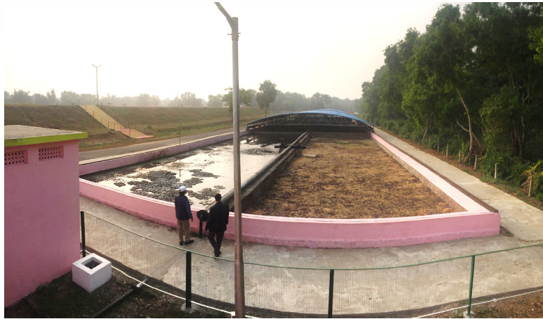
Figure 49: Proper Layout Planning of Sludge Drying Beds
