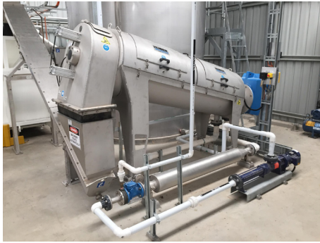
Figure 55: Mechanical Equipments at Site (Example of Ergonomics)
