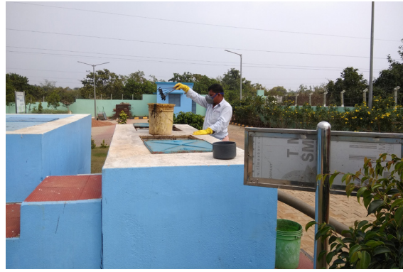
Figure 47: Enclosed Screen With Potential Hazard of Gases
