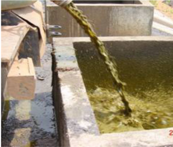
Figure 3: Picture of faecal sludge being emptied at a FSTP
