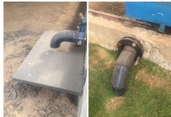
Figure 51: Use of Splash Plate To Reduce Erosion And Even Spreading of Sludge And Flange Joints For Easy O&M
