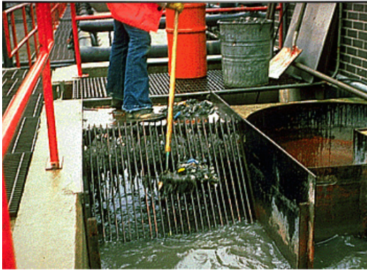
Figure 46: Screen Basket Without Adequate Access
