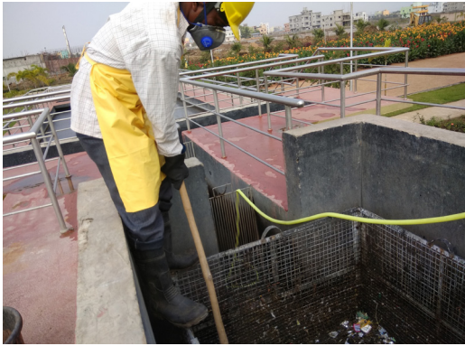
Figure 46: Screen Basket Without Adequate Access
