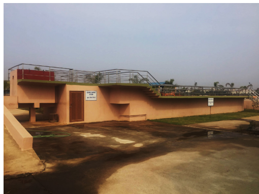
Figure 48: Safety rails | Easy access by road / pathway | Easy access to valves and pipes
