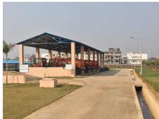
Figure 58: Adequate parking with good access by wide paved road Provision of storm water drains
